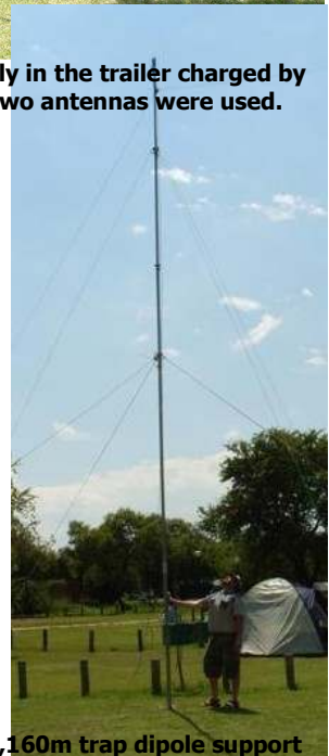
ZS6PJH checking the 40,80,160m trap dipole support
